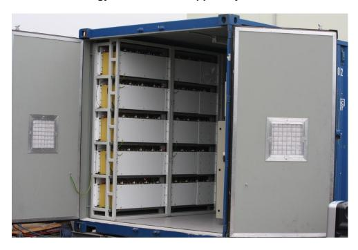
This version of GPSS-SWR comes with a solar charger which stores the solar energy in its batteries, and feeds this power back to the SWER network during periods of heavy loading.
