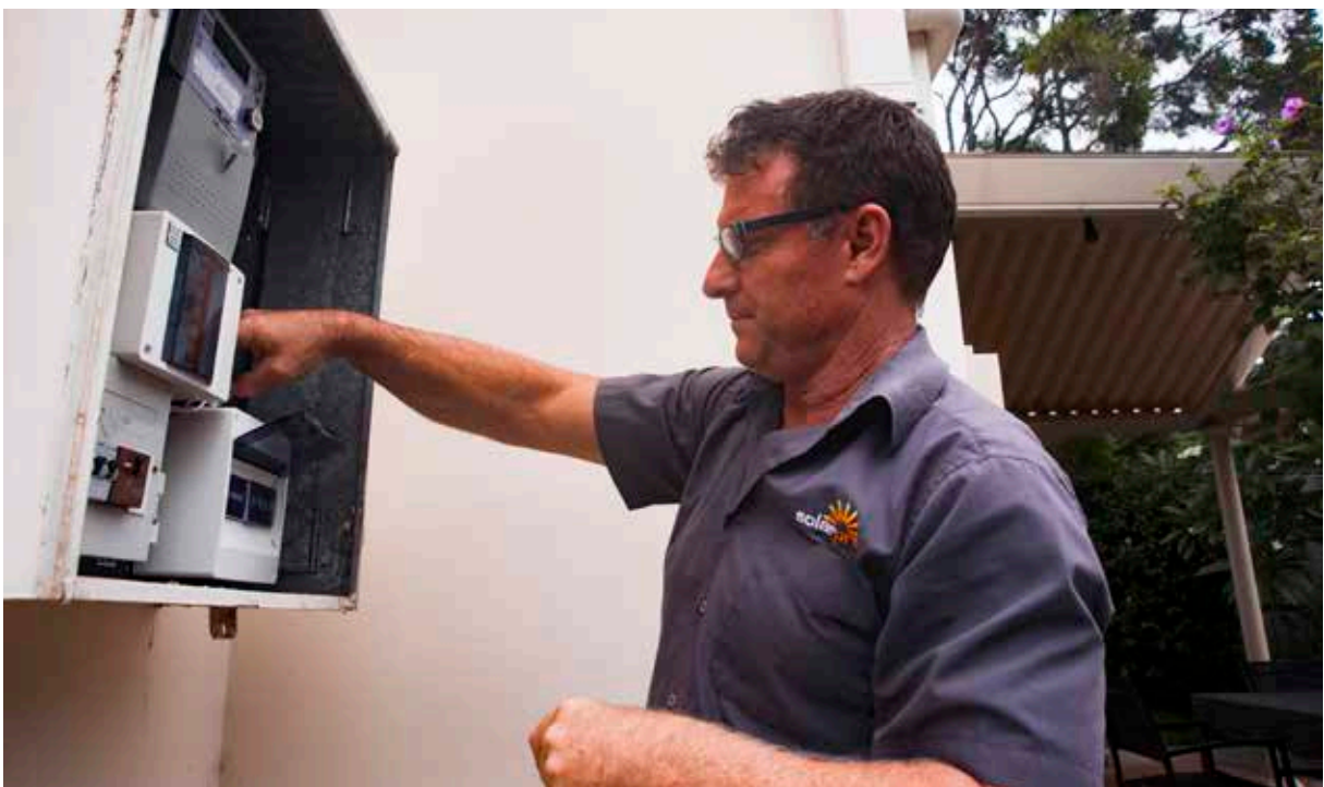
Photo courtesy Reposit Power
