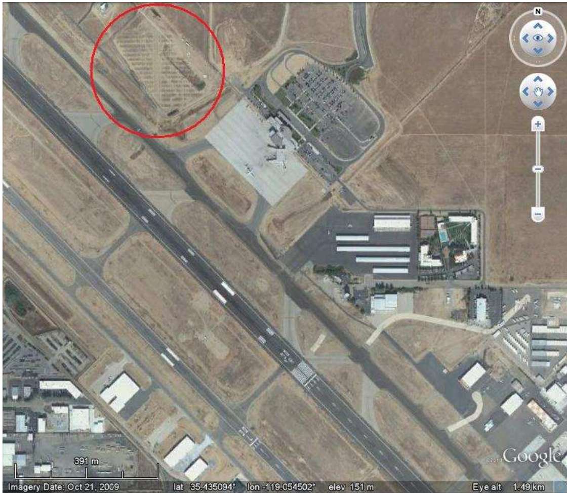
Figure 7: Bakersfield Airport showing location of solar array
