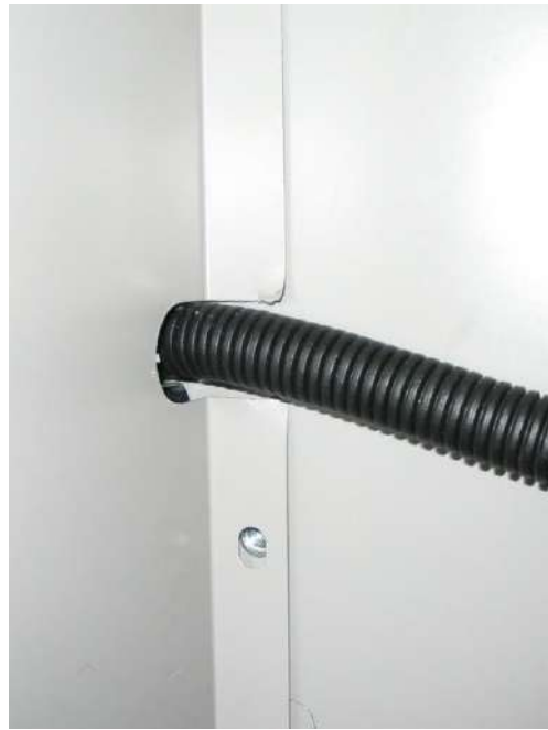
Step 16 remove the tab on the side of the electrical entry to the heat pump module
