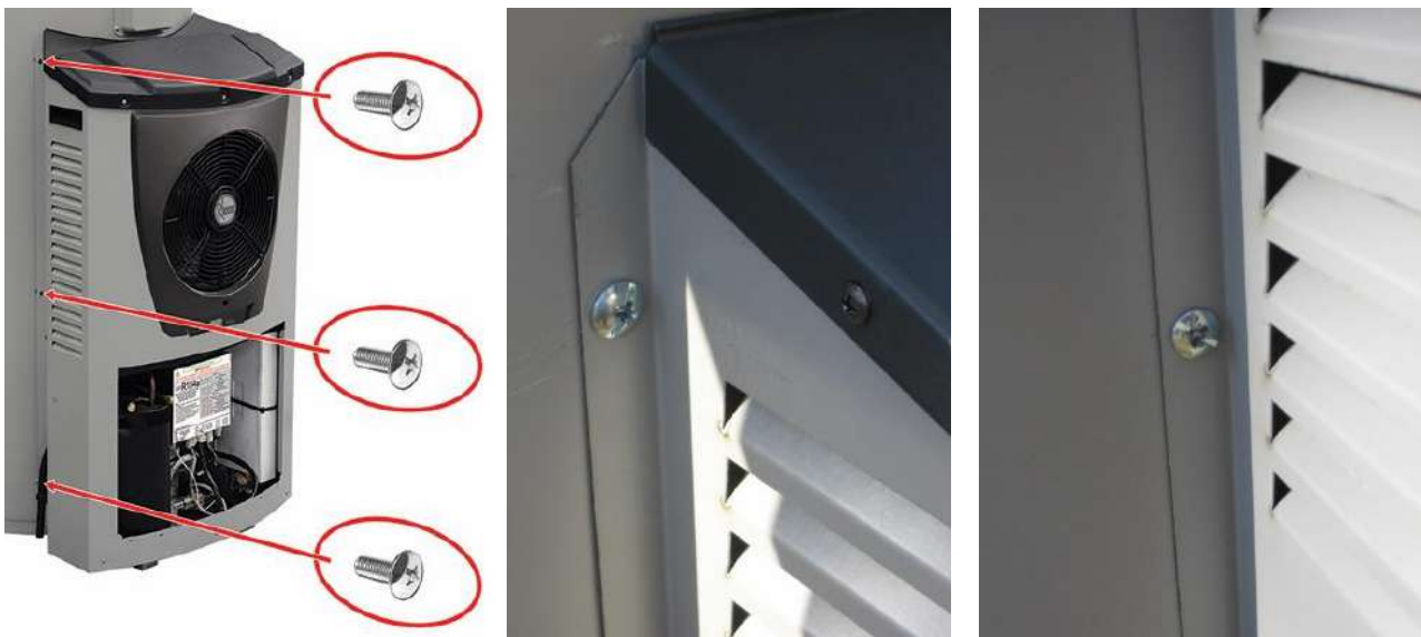
Step 21 screw in fixing bolts to connect heat pump module to storage tank
