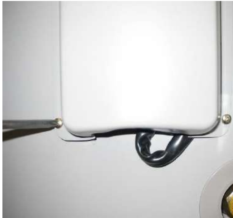
Step 2 remove screws from lower front cover
