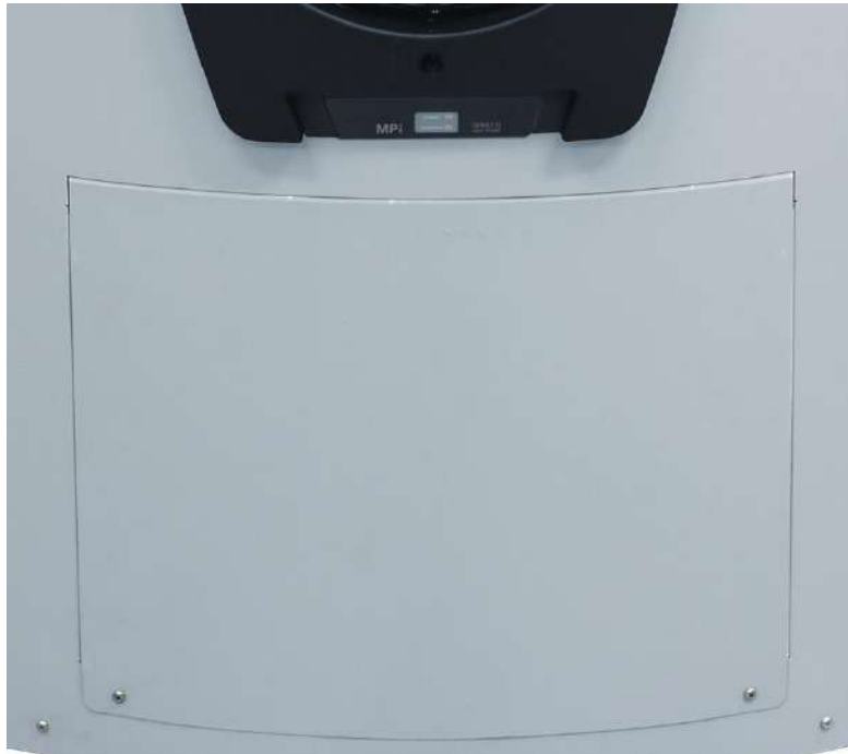
Step 27 replace heat pump module front cover
