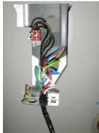
Step 3 withdraw the power cable
