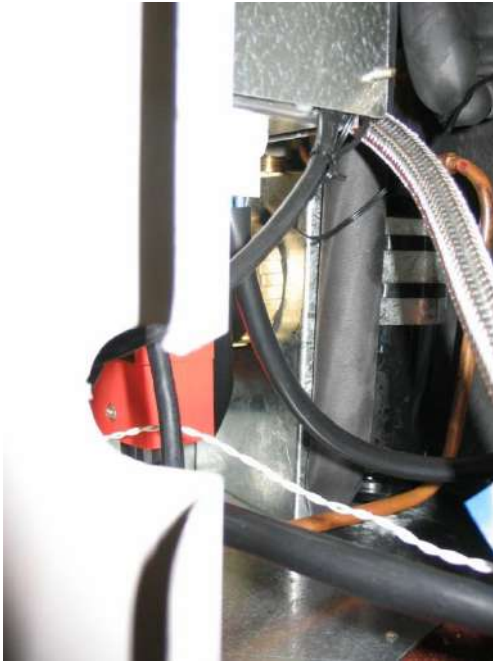
Step 16 remove the tab on the side of the electrical entry to the heat pump module
